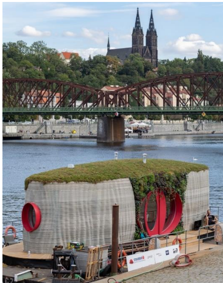
Fig. 5 The Prvok House after printing in the city center of Prague, Czech Republic (courtesy of Scoolpt s.r.o., adopted from [5]).
